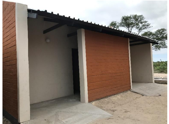
The new abluition block funded by the Japanese Government in order for the Mainstream Foundation to improve its hygiene management.
