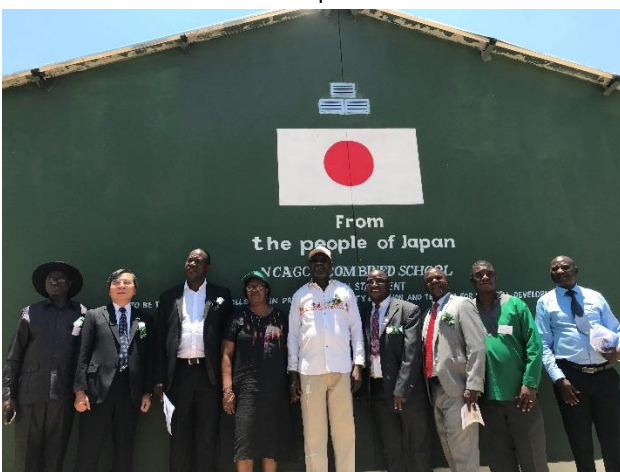
A Japanese flag was painted on the block constructed under the project, commemorating the contribution from the people and the Government of Japan
