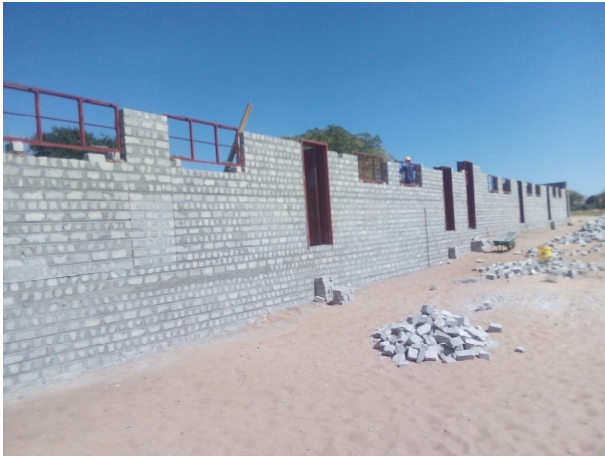
Photo of Ngwangwa Primary School's new classroom block taken on 7 May. Courtesy of Ngwangwa Primary School.
