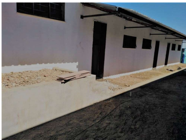
Photo of A.I. Steenkamp Primary School's new classroom block taken on 6 May. Courtesy of Directorate of Education, Arts and Culture, Khomas Regional Council.
