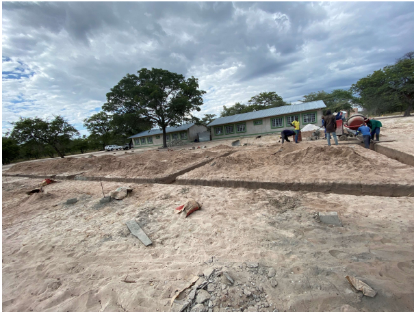
Photo of Egambo Combined School's new construction work taken on 11 May. Courtesy of Egambo Combined School.
