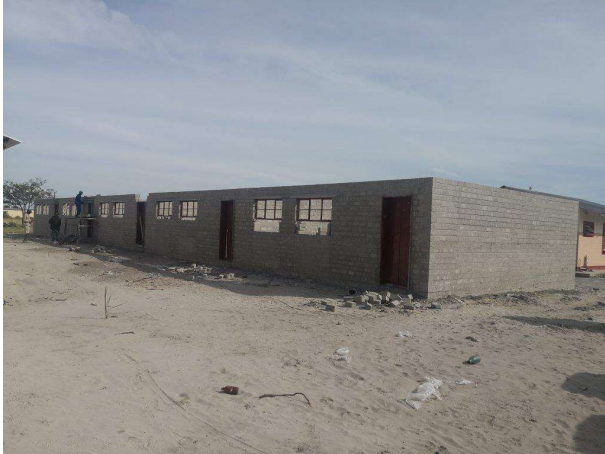
Photo of Kanono Combined School's new classroom block taken on 11 May. Courtesy of Kanono Combined School.
