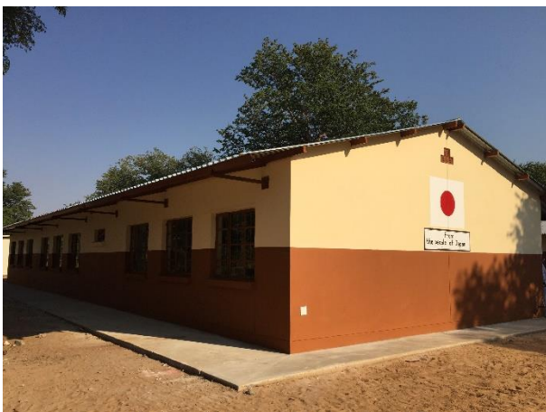
The new classroom block of Kaisosi Combined School
