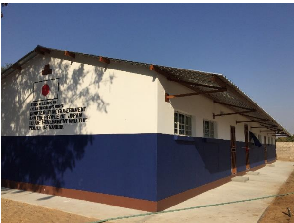
The new classroom block of Kehemu Primary School
