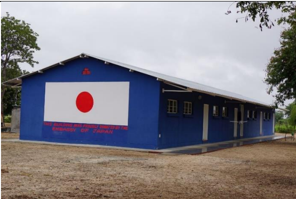
The new classroom block of David Shingo Combined School
