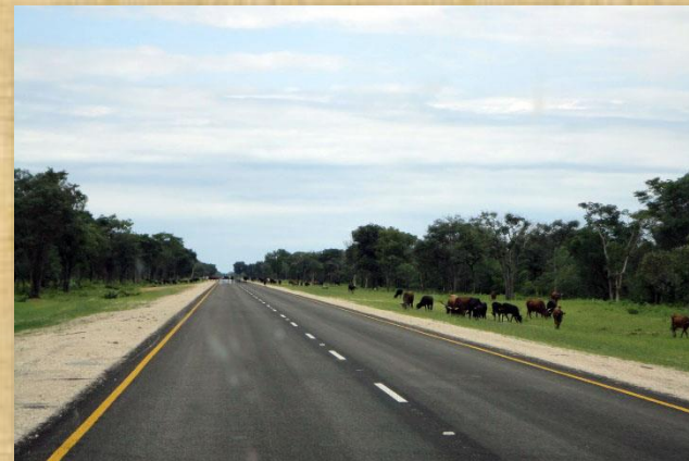
Rundu-Erundu (370km) road rehabilitation (L/A AUG 2006)
