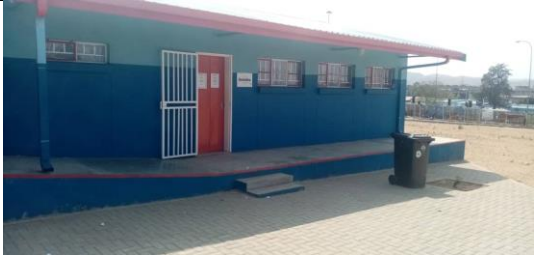
Photo 3: Constructed Library (Outside)
