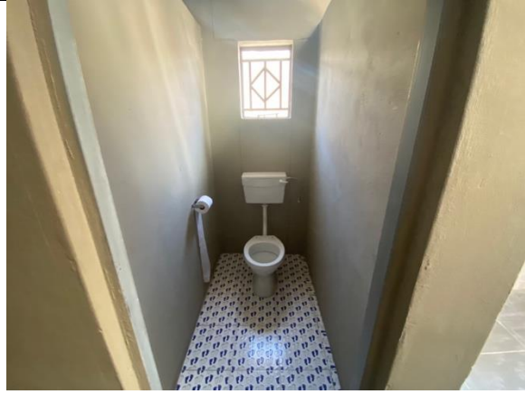
Photo 5: Constructed toilet at Savo Nuts Private School
