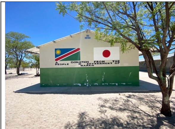
Photo 1: Constructed Classroom Block at Oipya Primary School
