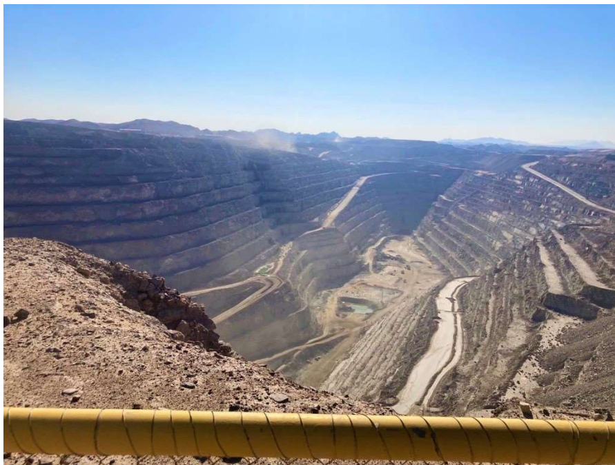
The SJ pit where mining has been conducted for the past 45 years. (3.5 km long, 1.5 km wide, and 420 meters deep)
